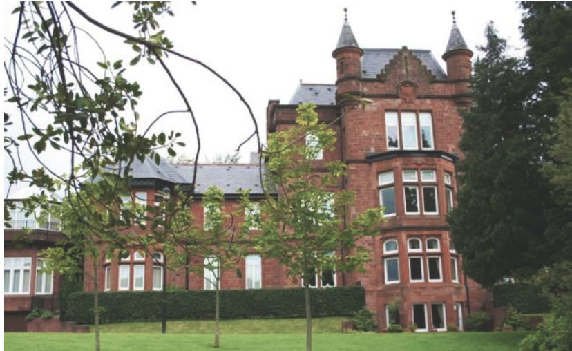
Redevelopment of the Former Bridge of Weir Hospital
